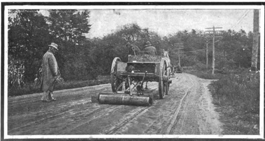
The small road roller and drag that are used in preparing roadbeds for their top dressing
